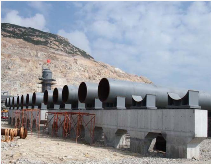
Liwan Slug Catcher Finger Installation
