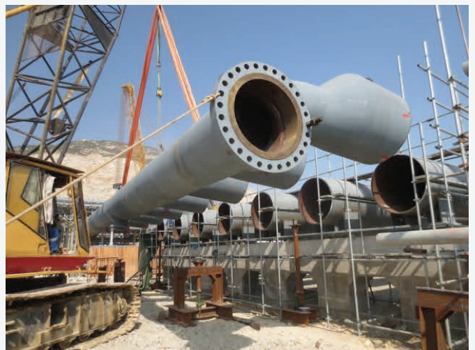
Outlet Liquid Header Being Installed (1 of 4)
