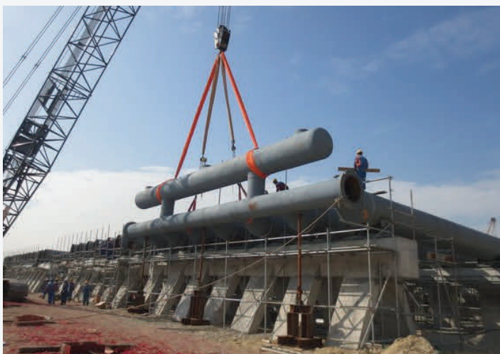
Primary Inlet Liquid Header Being Installed (1 of 4)
