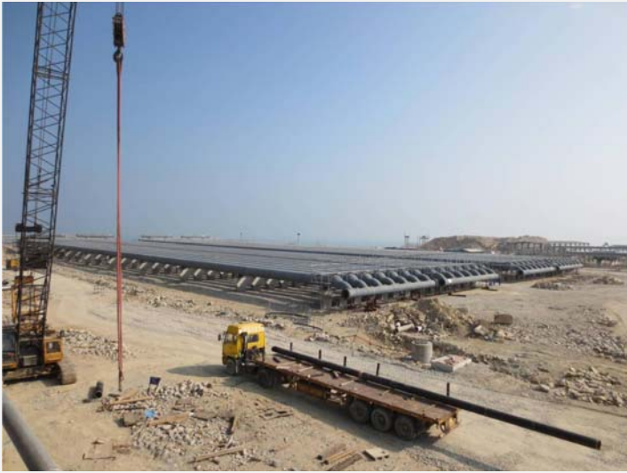
Liwan Slug Catcher Nears Completion
