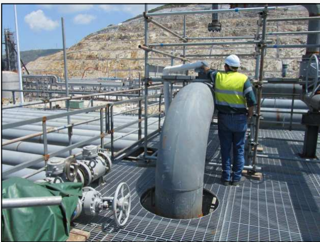
Slug Catcher being prepared for Hydro Testing
