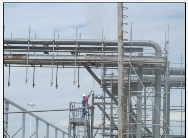
Pressure being relieved after 10 min. of testing
