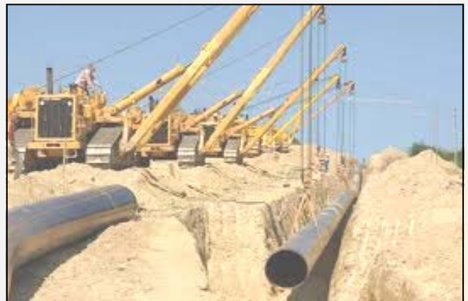
A Natural Gas Pipeline Under Construction in the United States
